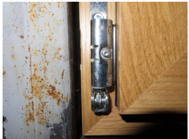
Picture 6 Hinge seen from opening side, inactive casement at bottom
