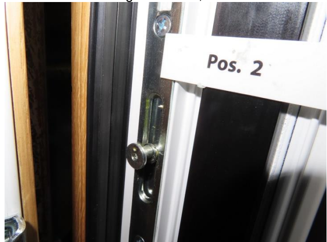
Picture 22 Locking situation 1, casement
