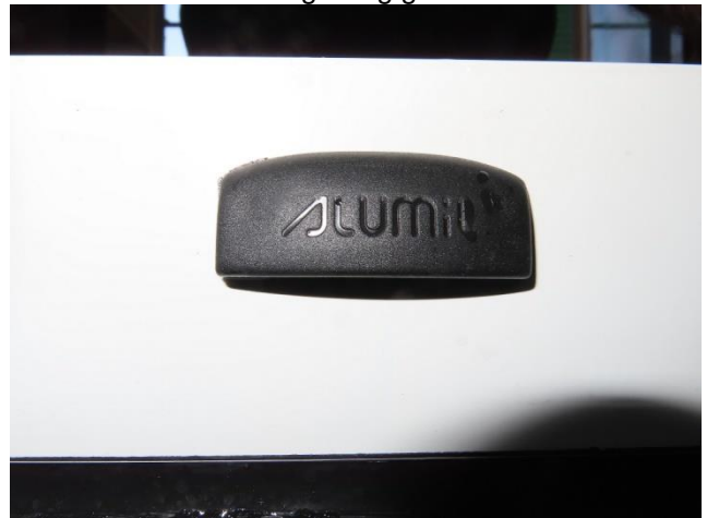
Picture 18 Drainage slot, seen from outside
