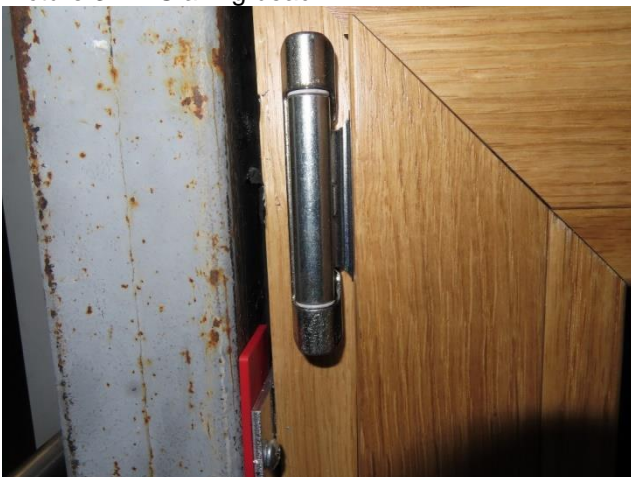
Picture 5 Hinge seen from opening side, inactive casement at top
