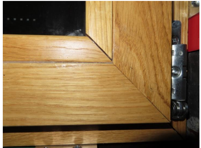
Picture 8 Hinge seen from opening side, active casement at bottom
