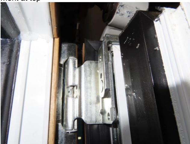
Picture 11 Hinge seen from rebate, active casement at top
