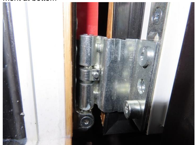
Picture 12 Hinge seen from rebate, active casement at bottom
