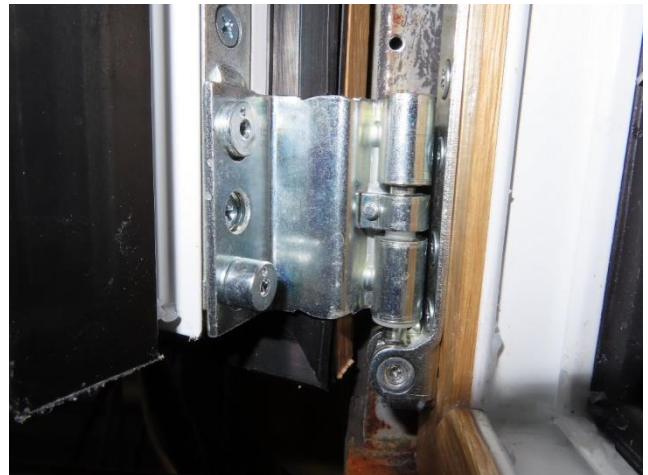
Picture 10 Hinge seen from rebate, inactive casement at bottom
