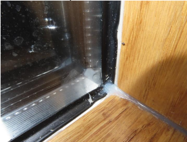
Picture 15 Internal glazing gasket
