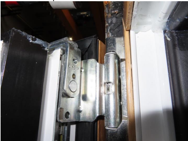
Picture 9 Hinge seen from rebate, inactive casement at top
