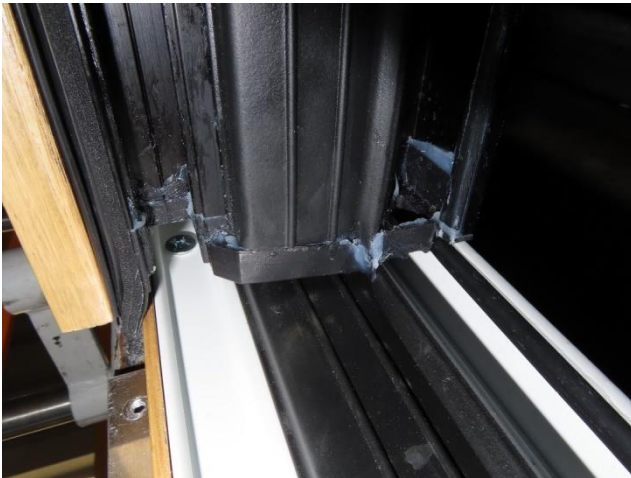
Picture 13 Dummy mullion at bottom
