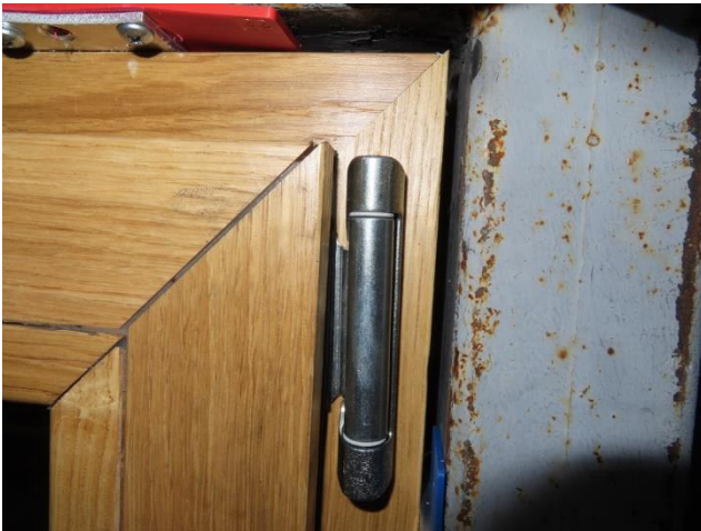
Picture 7 Hinge seen from opening side, active casement at top
