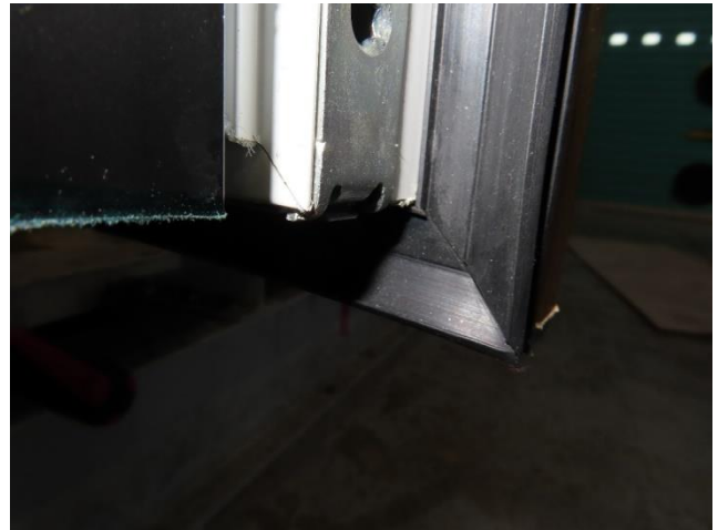
Picture 14 Casement seal at bottom
