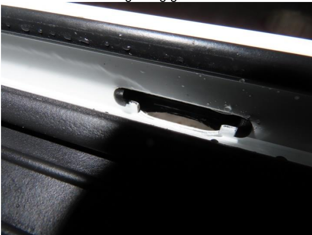
Picture 17 Frame at bottom with rebate drainage slot
